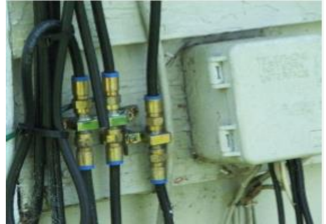
(a) Coaxial Cable-simple joints
